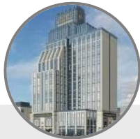
GCP Surawong (Under Development)
