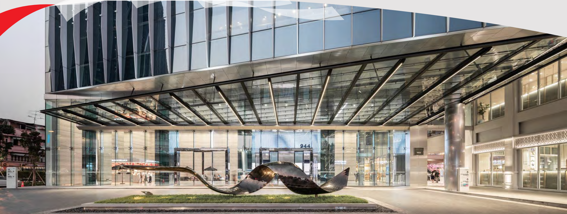
Mitrtown Office Tower, Bangkok | Thailand
